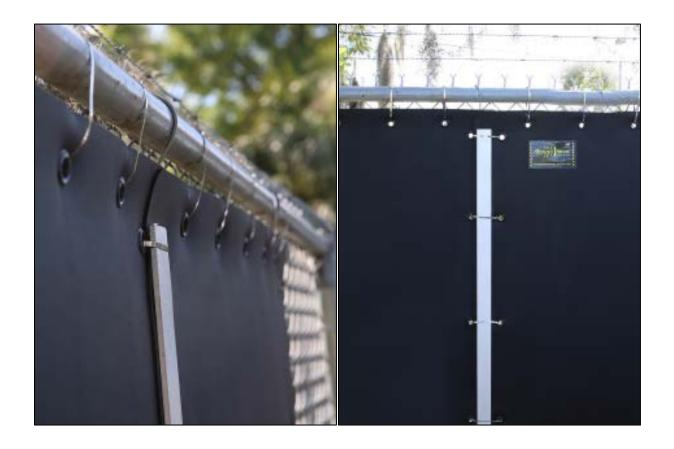
Another option is adding a 1.5" wide x ¼" thick metal bar to the seam. This will significantly strengthen the seam as well as closing much of the air gaps in the seam, which allows sound penetration. When the zip ties are cinched it sandwiches the 2 layers of AcoustiFence between the metal bar and the chain link fence. The metal bar could also be taller than the AcoustiFence section, with one end buried into the ground so that the bottom edge cannot move.
